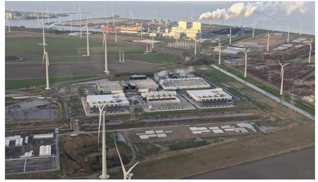
Aerial view of the Google data center at Eemshaven, Netherlands, surrounded by wind turbines and a nearby power plant. As AI expands, data centers like this require large amounts of electricity, making energy supply a key challenge. Photo by Wvdp (Wikimedia Commons).
