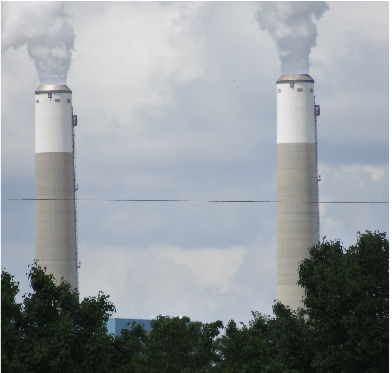
Stacks of Clover Power Station in Clover, Virginia, United States, a coal-fired plant whose retirement has been postponed until 2045 as electricity demand grows with the expansion of AI-related data centers. The delay is part of a wider pattern in which older coal facilities are being kept in service to support rising power needs from digital infrastructure. Photo by Emw (Wikimedia Commons).
