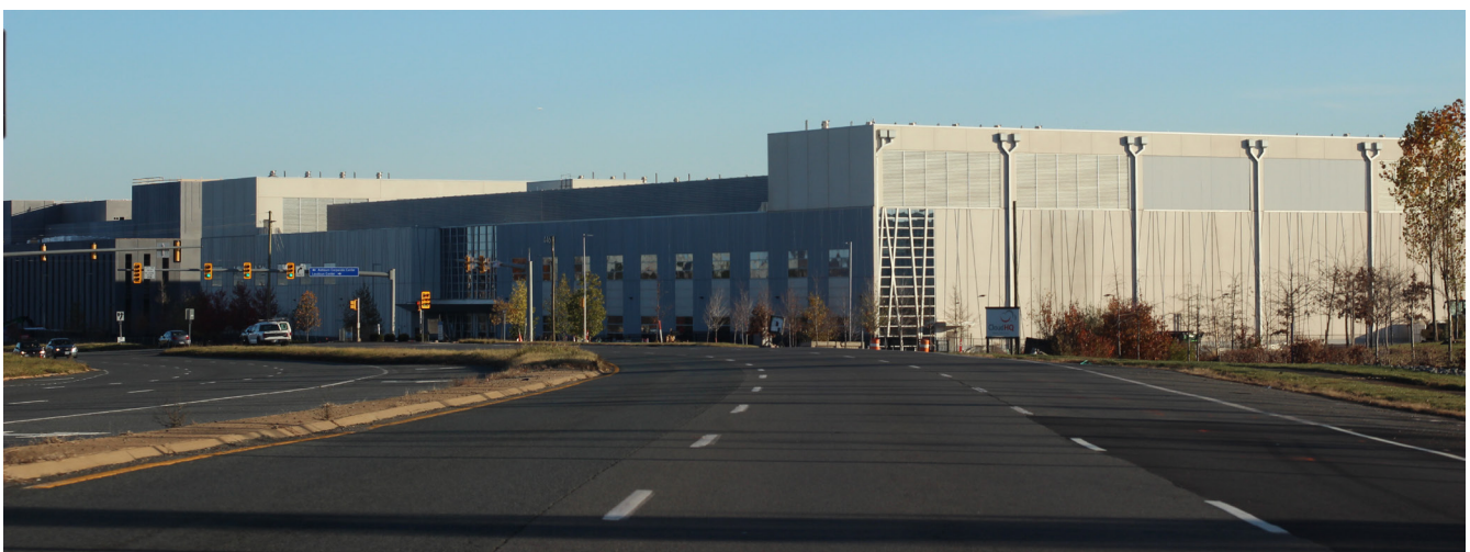
Data center in Ashburn, Virginia, United States. One of the world's largest concentrations of data centers, the area hosts dense clusters of facilities powering global cloud and AI services, underscoring how digital infrastructure is concentrated in a few regions amid a widening global divide. Photo by Emily Richardson (Flickr).
