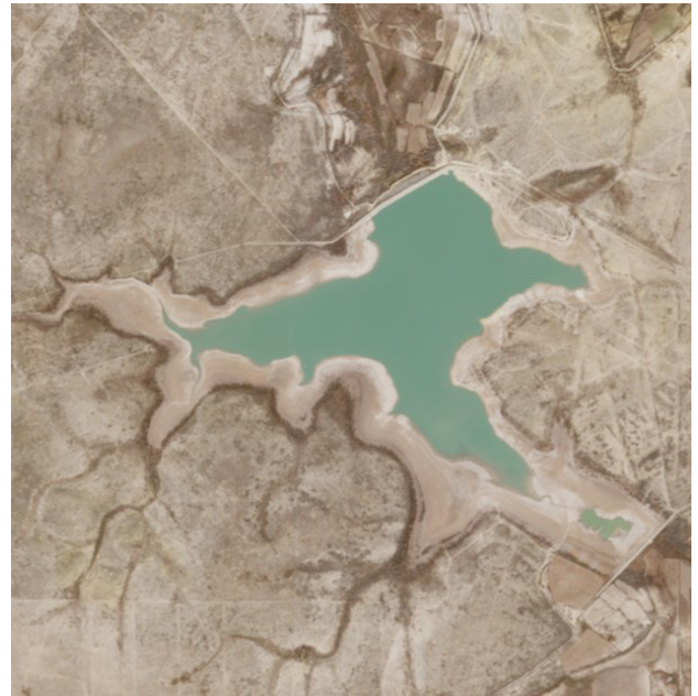
Aerial view of Presa El Centenario reservoir in Querétaro, Mexico—known as the country’s data center capital—where prolonged drought has sharply reduced the reservoir’s surface area. Yet, expanding AI data centers in the region are drawing on limited water supplies for cooling and energy production, intensifying pressure on communities already facing water shortages. Data source: Sentinel-2 imagery, February 2026.
